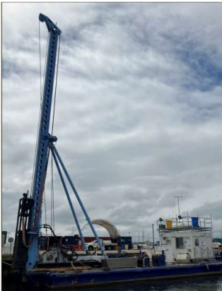
Figure 2: 18m pile driving barge utilised for works
